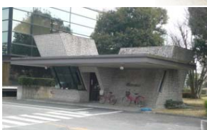
The gate station is designed to express the left and right blade setting
