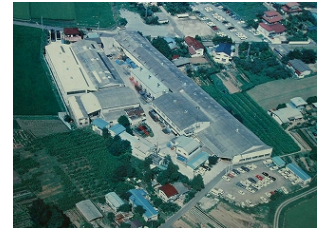
Amada Engineering / Fukushima Plant
