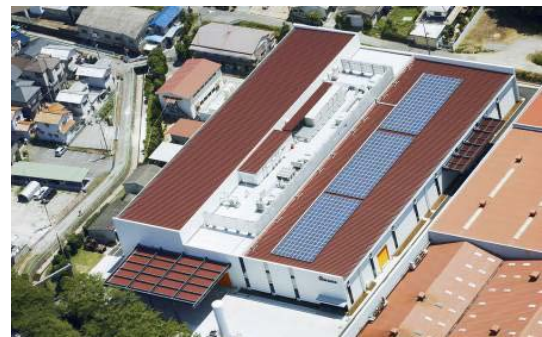
Solar panels at Ono Plant
