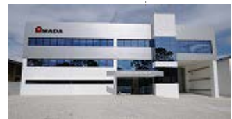
Technical Center in São Paulo (Brazil)
