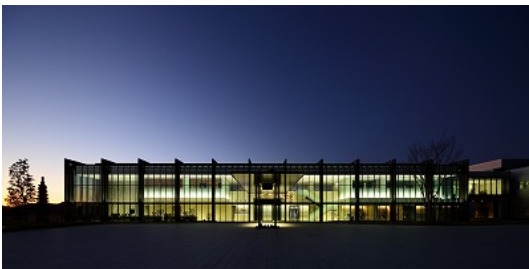
Toki Works Technical Center lighting
