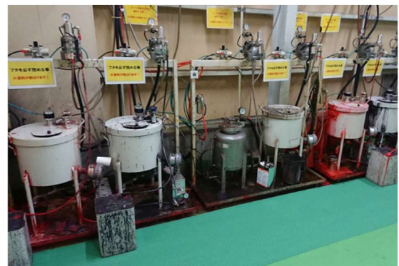
Solvent paint mixing room (Fukushima Plant)
