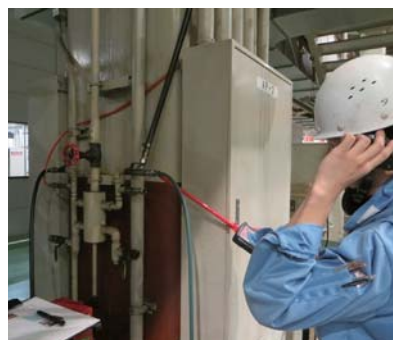
Air leak patrol (Fujinomiya Works)
