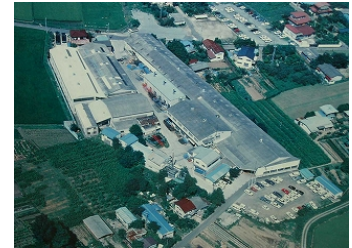
Amada Automation Systems / Fukushima Plant
