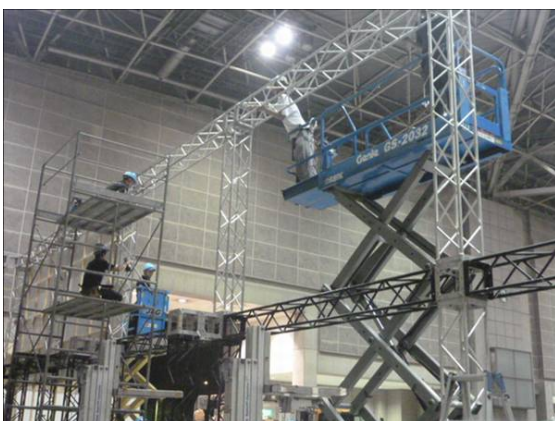
Framework construction at the MF-Tokyo exhibition. Construction components are reused.
