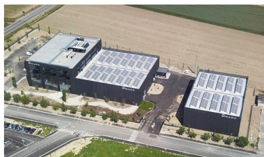
Amada Italy’s solar panels
